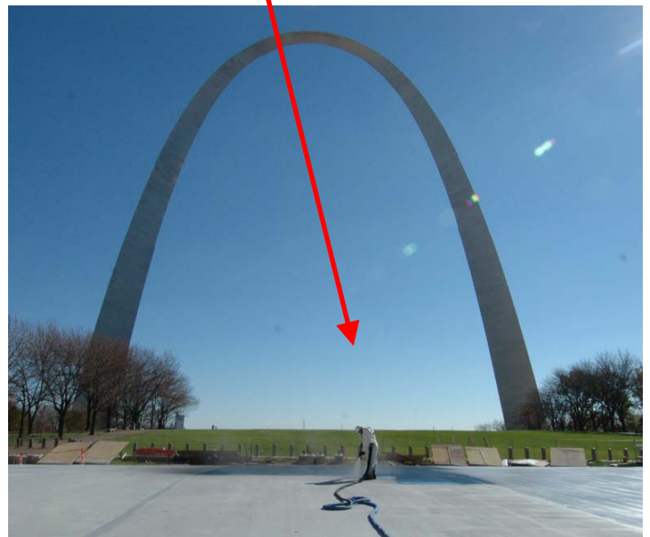
APPLICATION OF FAST SET POLYUREA SYSTEM
