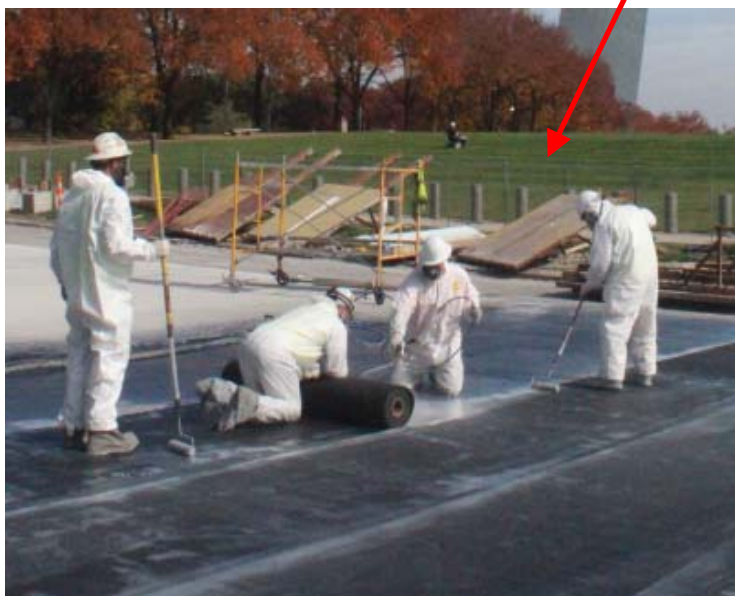
APPLICATION OF 5 MINUTE CURE POLYURETHANE SYSTEM WITH REINFORCING GEOTEXTILE FABRIC
